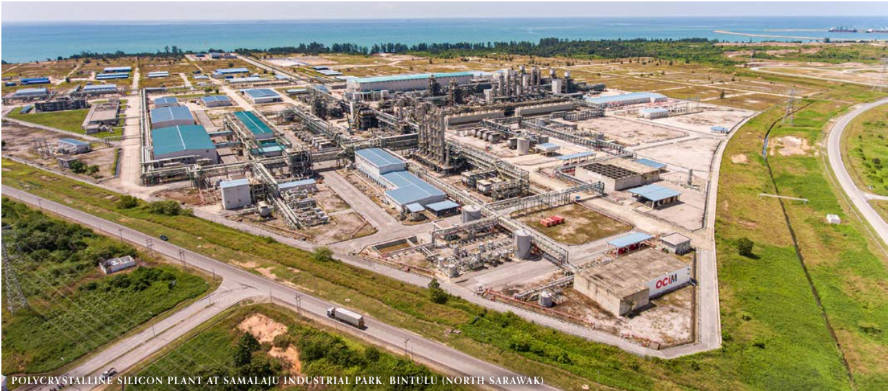
POLYCRYSTALLINE SILICON PLANT AT SAMALAJU INDUSTRIAL PARK, BINTULU (NORTH SARAWAK)
